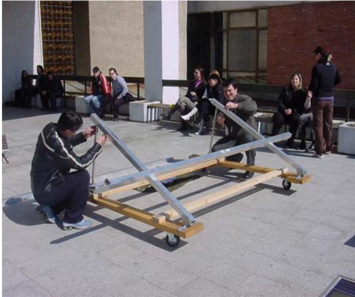
Fig. 3 The laboratory exercise “Mountaing the PV rack”.
